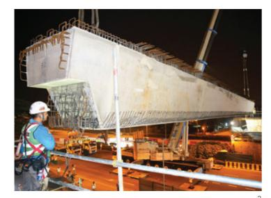
"We couldn't interrupt 'live' airport operations and had to coordinate the diversions of all incoming and outgoing traffic onto one carriageway, so that we could raise the structure. This was done within a time-frame of four hours each night, over eight nights," she recalls.
